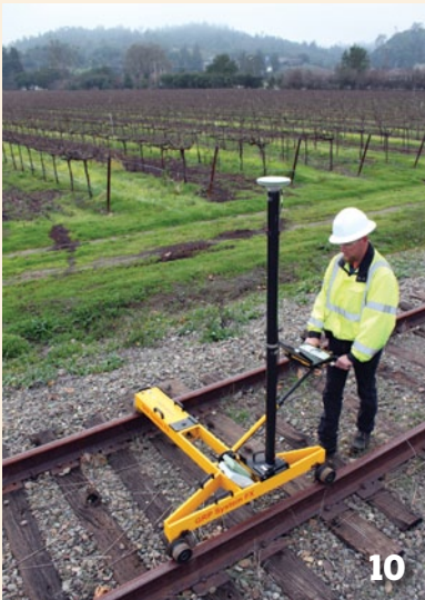
10 James Brown of Cinquini & Passarino (Santa Rosa, CA) uses the Amberg GRP to gather track geometry for the Sonoma-Marin Area Rail Transit project.
