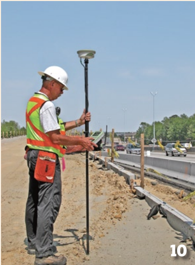
John F. Hill, Jr., LS of Alphatec Surveyors surveys a major transportation project in Chesapeake, VA with a Leica SmartRover connected to Loyola's RTK-Net.
