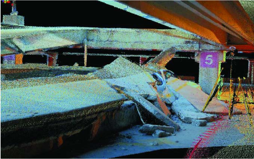
Combined scan/orthophoto detail of floor of CAMC parking garage
