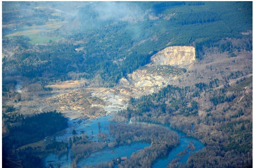
An aerial view of the Stillaguamish River and State Route 530 after the Oso landslide on March 22. The landslide resulted in the damming of the Stillaguamish River in Snohomish County. Mud covering the area, including SR 530, is a mile wide.
