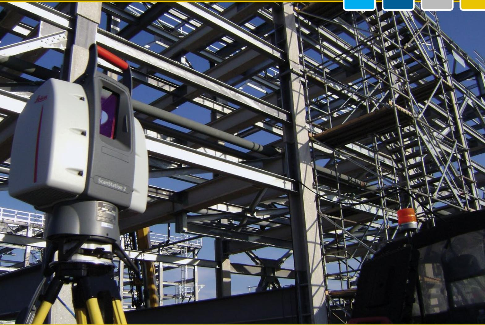
Cianbro surveyors use high definition scanner to create measurable 3D digital images that are then used to verify component positional accuracy.
