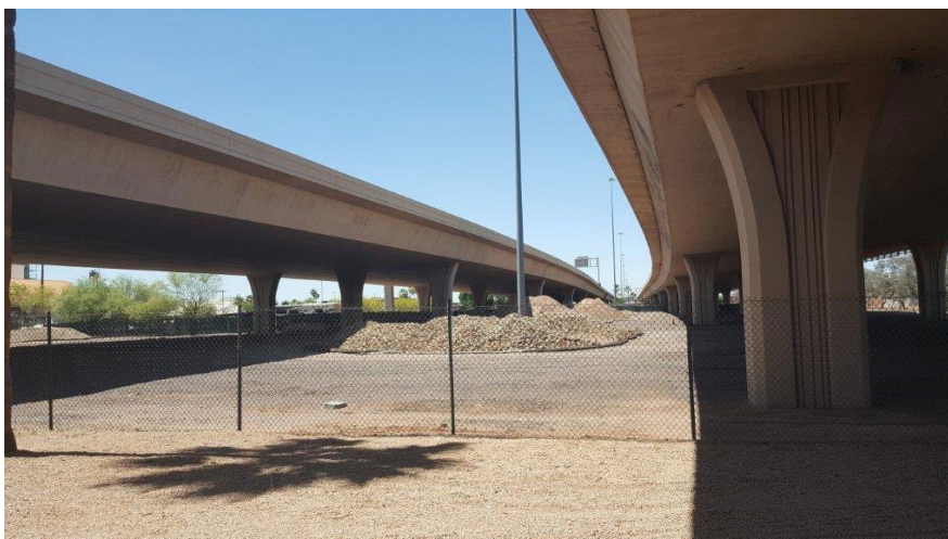
Interstate 10 and 15th Avenue (Althea Street) occupies the site of this monumental boundary case. Google Earth coordinates are 33°27'42.20 N and 112°05'30.17"W.
